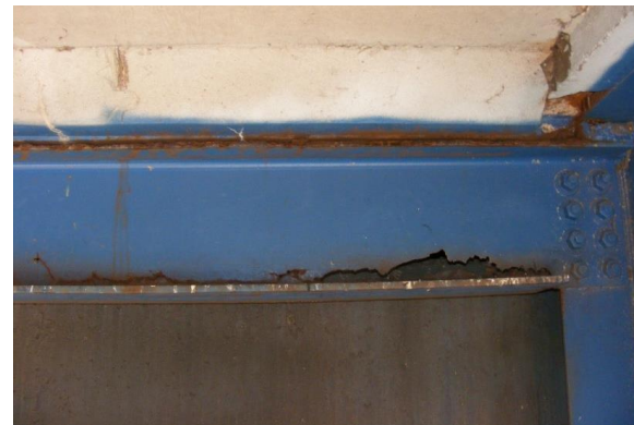
Figure 12 [Beam Corrosion]
