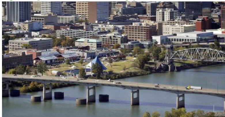
Figure 10 [I-30 Arkansas River Bridge]
